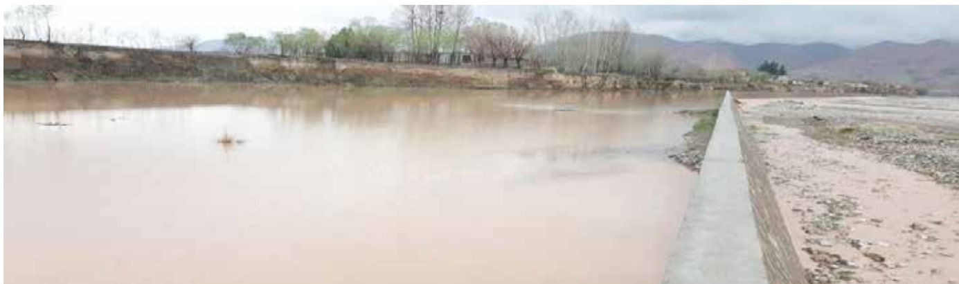
Water Ponding Behind the Retaining Wall
