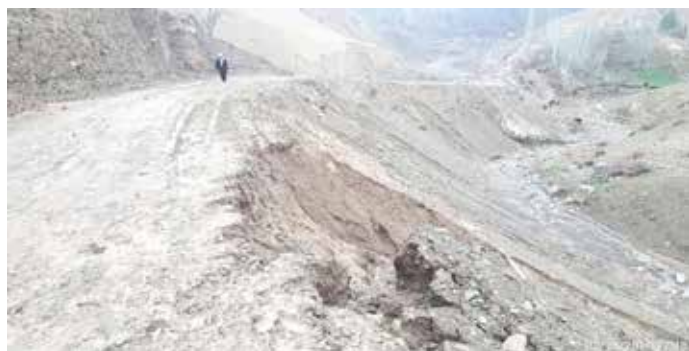
Slope Collapse
