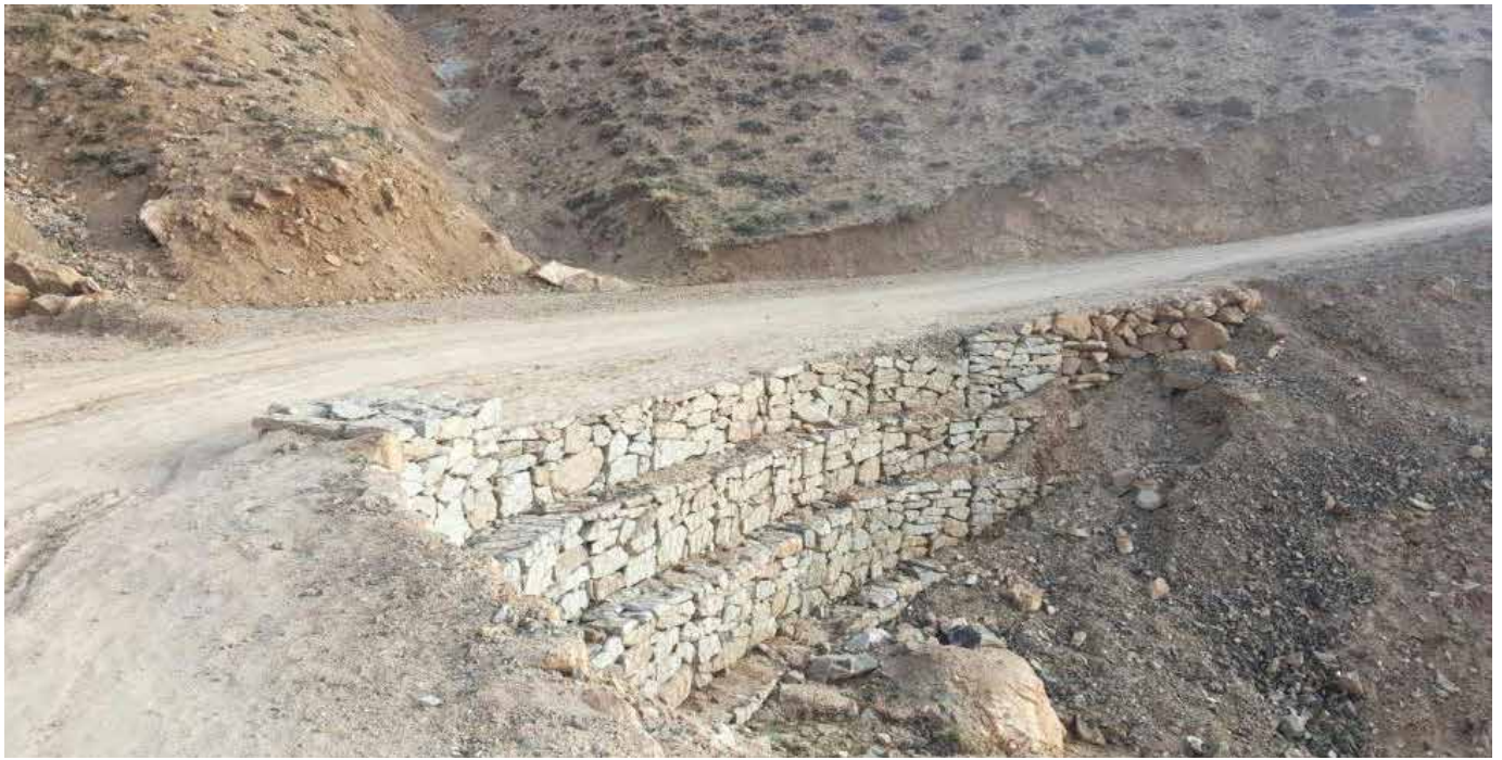
Retaining Structure along Waras Rural Road
