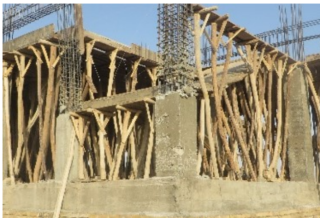
Figure 23: Improper formwork and lack of spacer usage caused uncovering of steel bars at the parapet walls.
