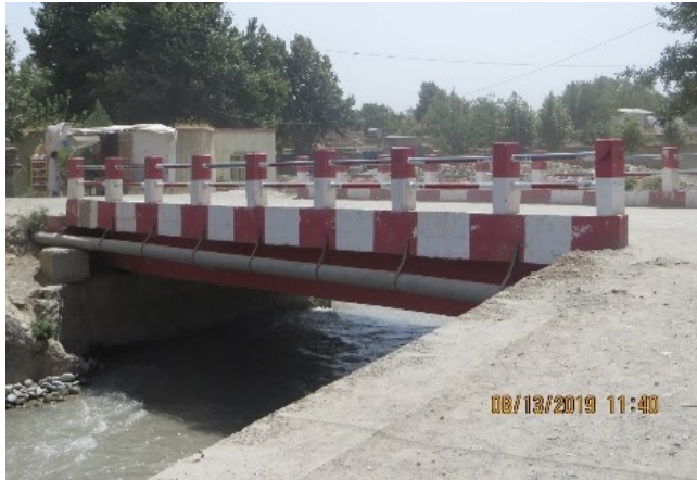
Figure 13: Construction of 12-meters Concrete bridge, Takhar Province
