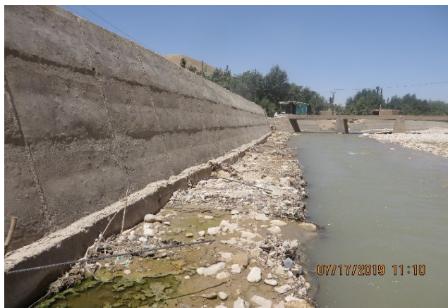
Figure 18: poor formwork was observed throughout the scheme wall
