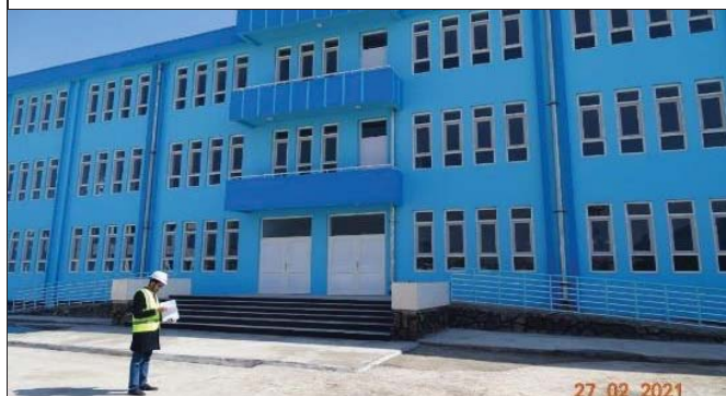
The assurance report team member during project site visit
