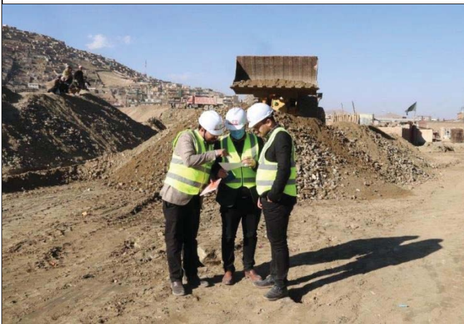
The assurance team members during site visit
