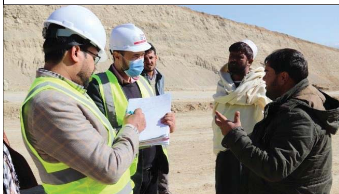
The assurance team members during site visit
