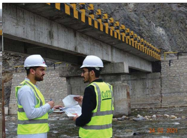
The assurance team members checking project RFQ and project specification with the project site
