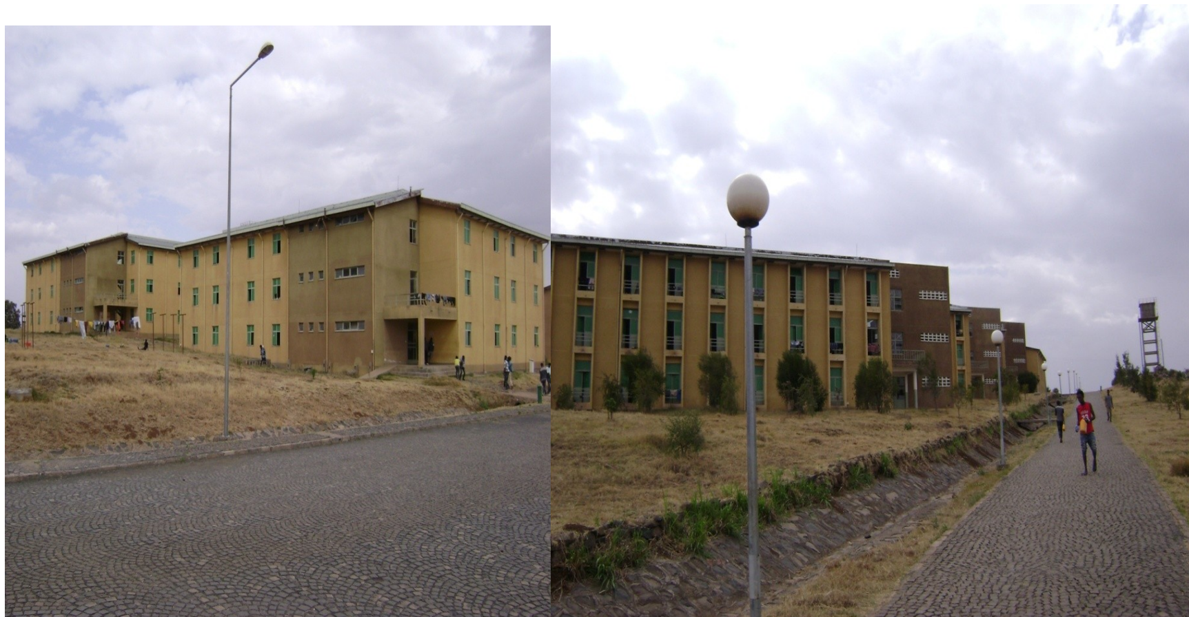
Figure 2-Dormitories (CYT+DHB Buildings) & Road Section (Infrastructure)
