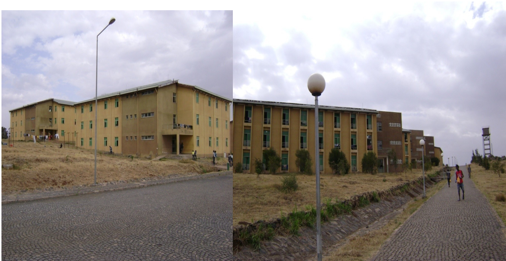
Figure 2-Dormitories (CYT+DHB Buildings) & Road Section (Infrastructure
