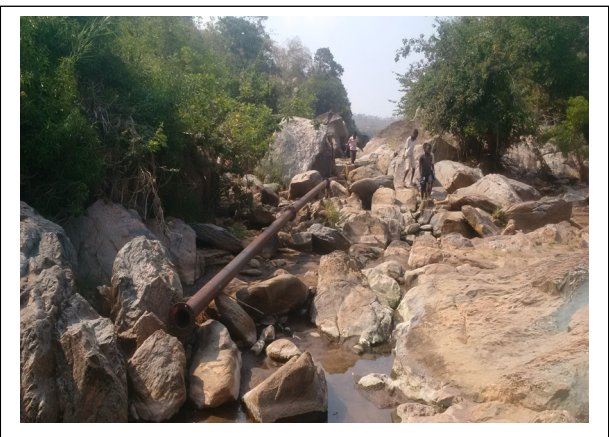
New Intake silted and abandoned
