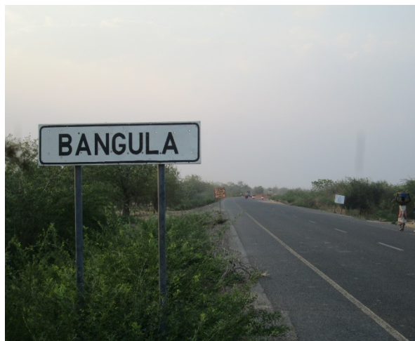
Section of Bangula – Nsanje Road at Bangula
