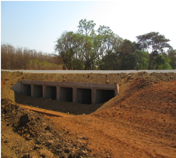
Six Cell Box Culvert
