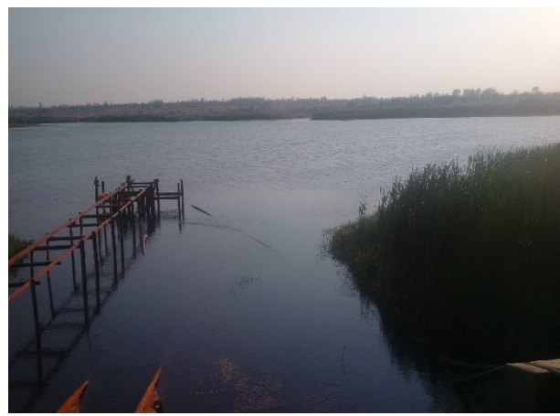
Nguluyanawambe Intake Structure
