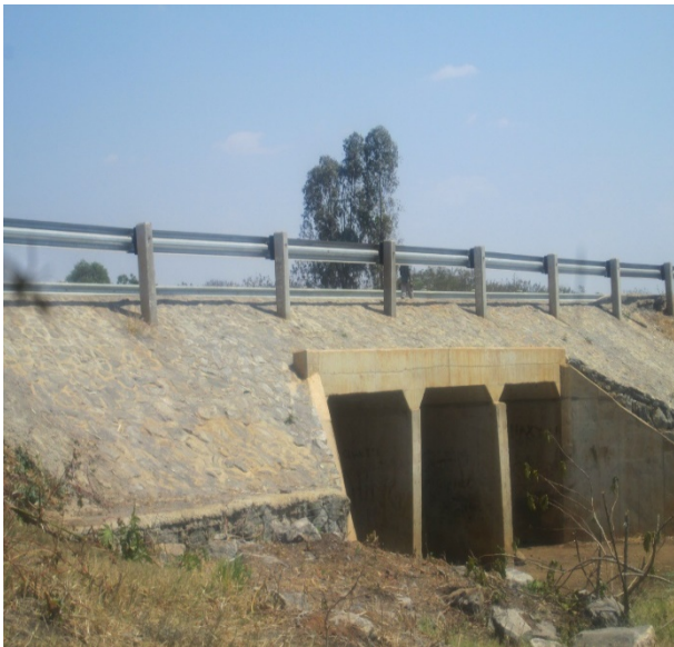
Three Cell Box Culvert near Bunda Junction
