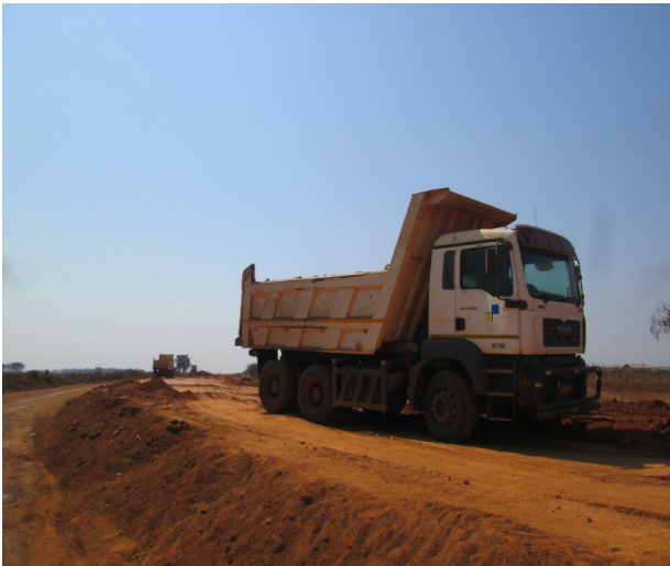
Earthworks in Progress
