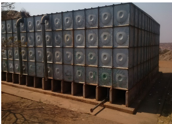
Refurbished water tank at Ngwenya
