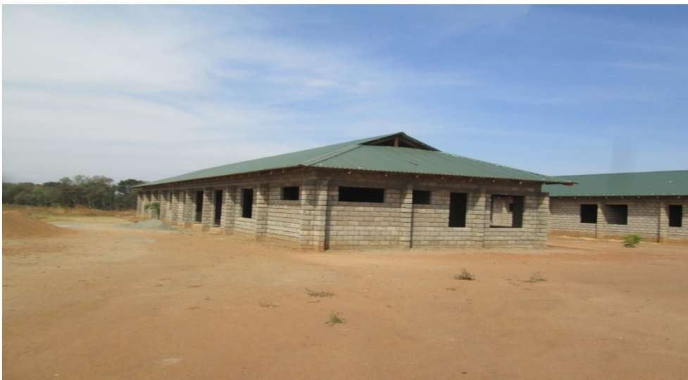
Domasi Rural Hospital Project – Abandoned incomplete Buildings
