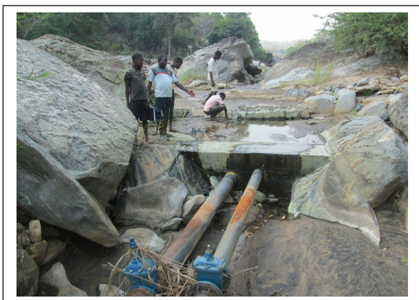
New Intake silted and abandoned
