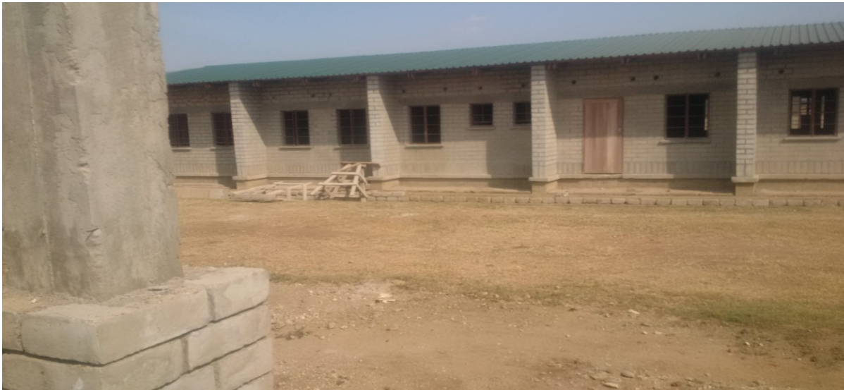
Machinga Secondary School – Incomplete Classrooms
