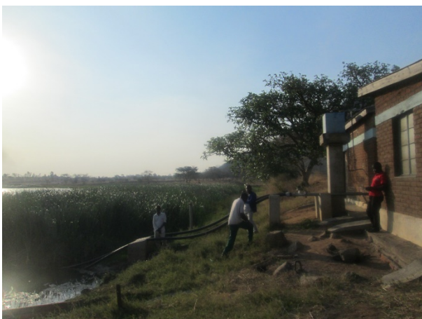
Nguluyanawambe Intake Pump House
