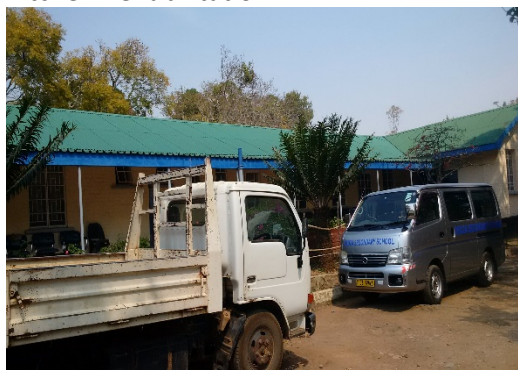
Administration Block – Rehabilitation
