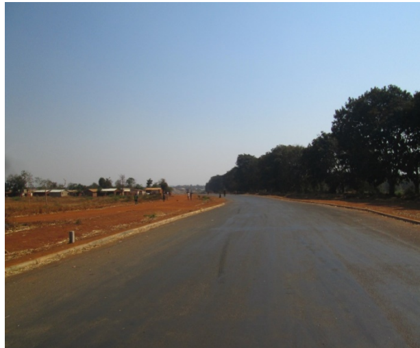
Completed Section near Mchinji Road Junction
