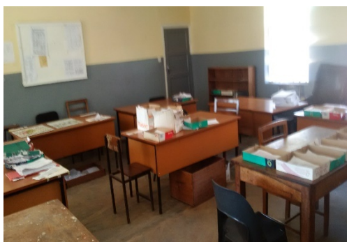
Staff Room – Rehabilitation
