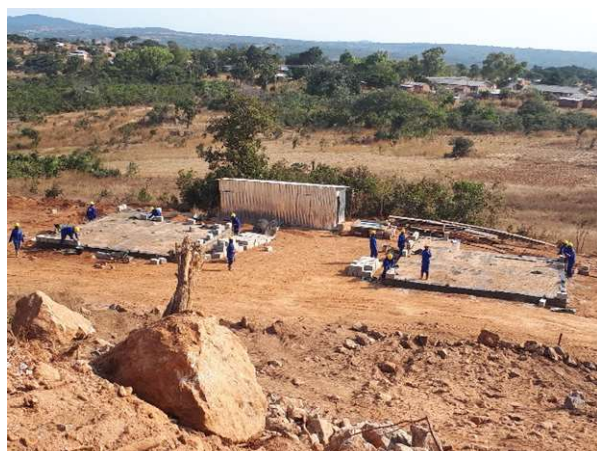
Picture 4.10.3 – Housing foundations at Kazomba Hill
