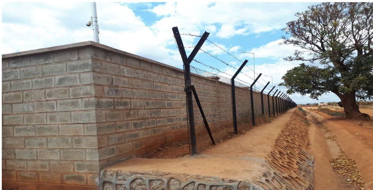
Photo 4.3.2 – New Fence at NOCMA Yard
