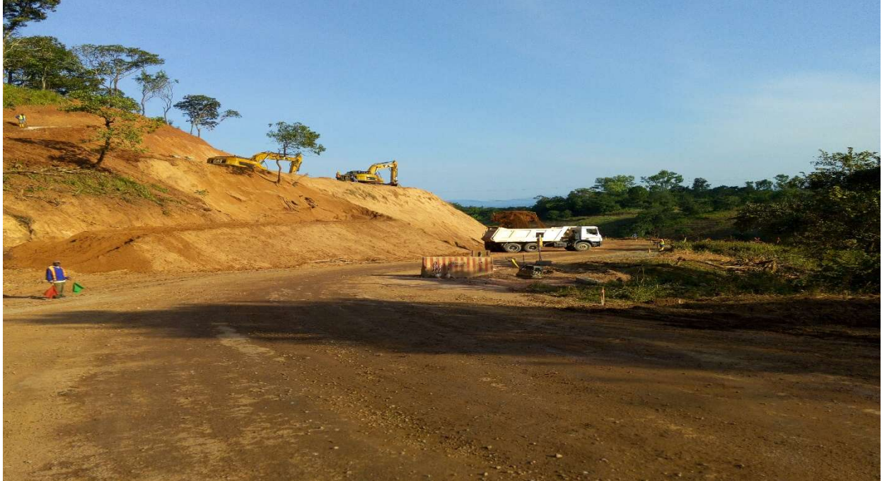
Picture 4.4.4.1 – Benching Slope Protection against Earthworks Collapse
