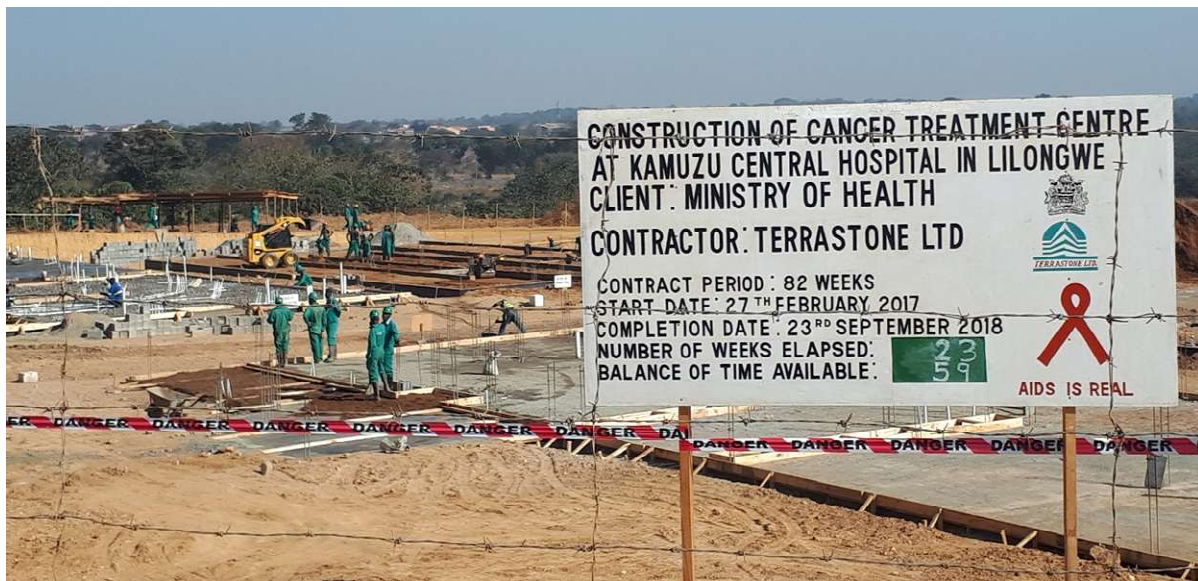
Photo 4.2.2.3 – Foundation works under construction
