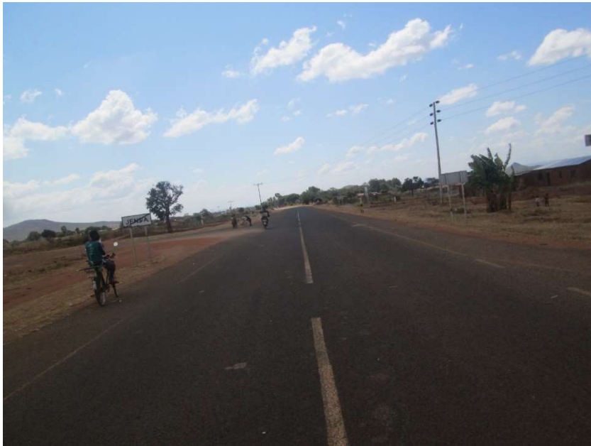
Picture 4.4.2.1 – Section of the Road near Jenda
