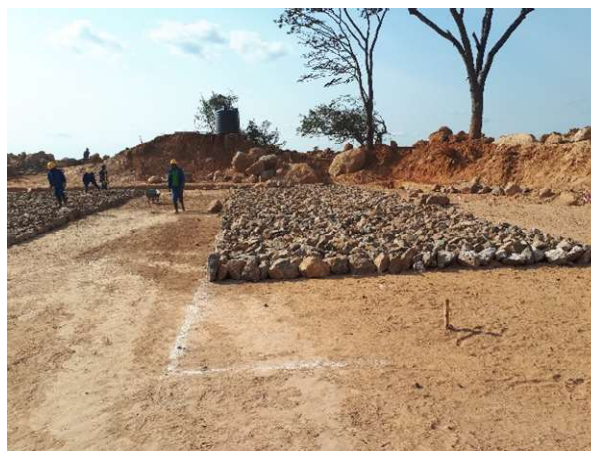
Picture 4.10.4 – Water Tank Foundations at Kazomba Hill
