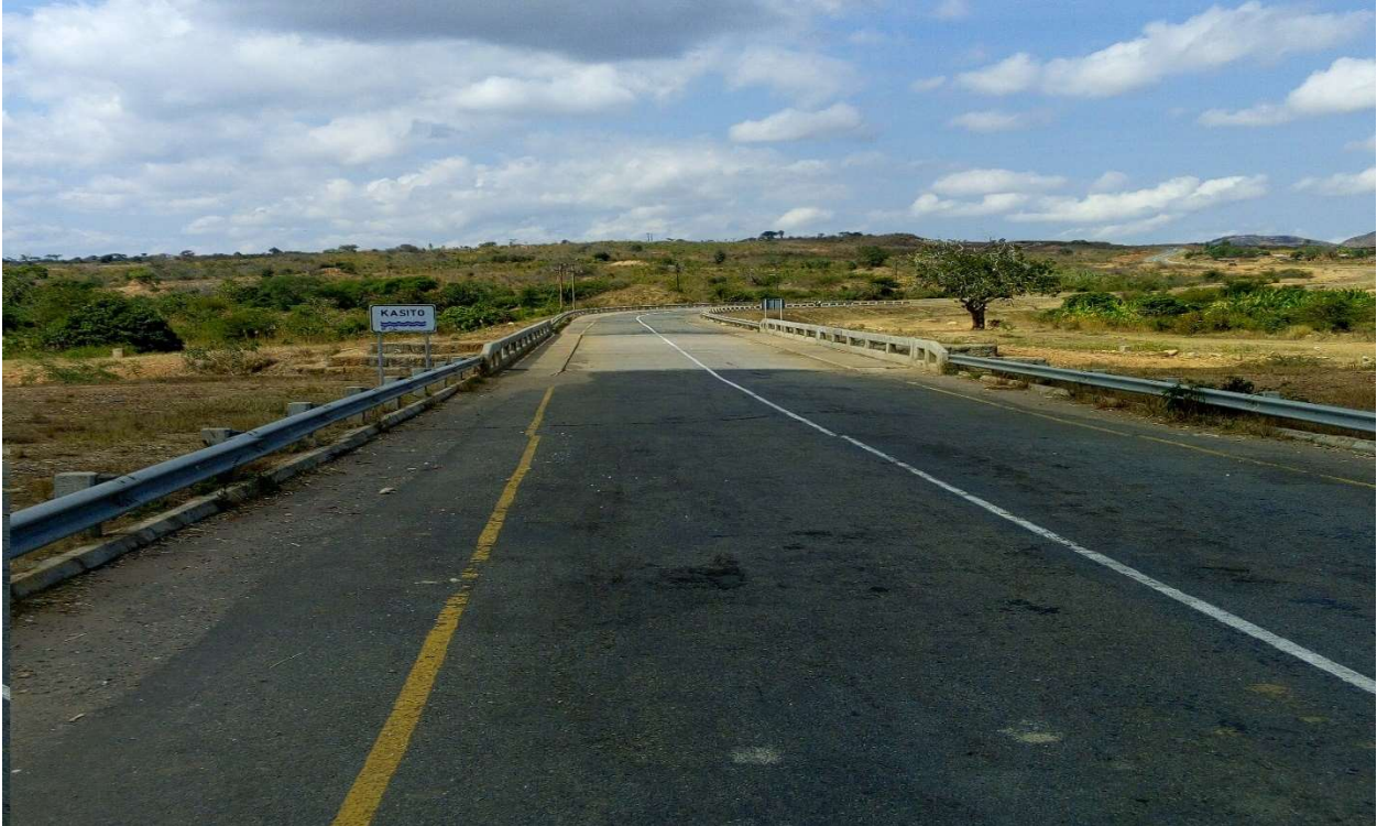
Road Section at Kasito Bridge
