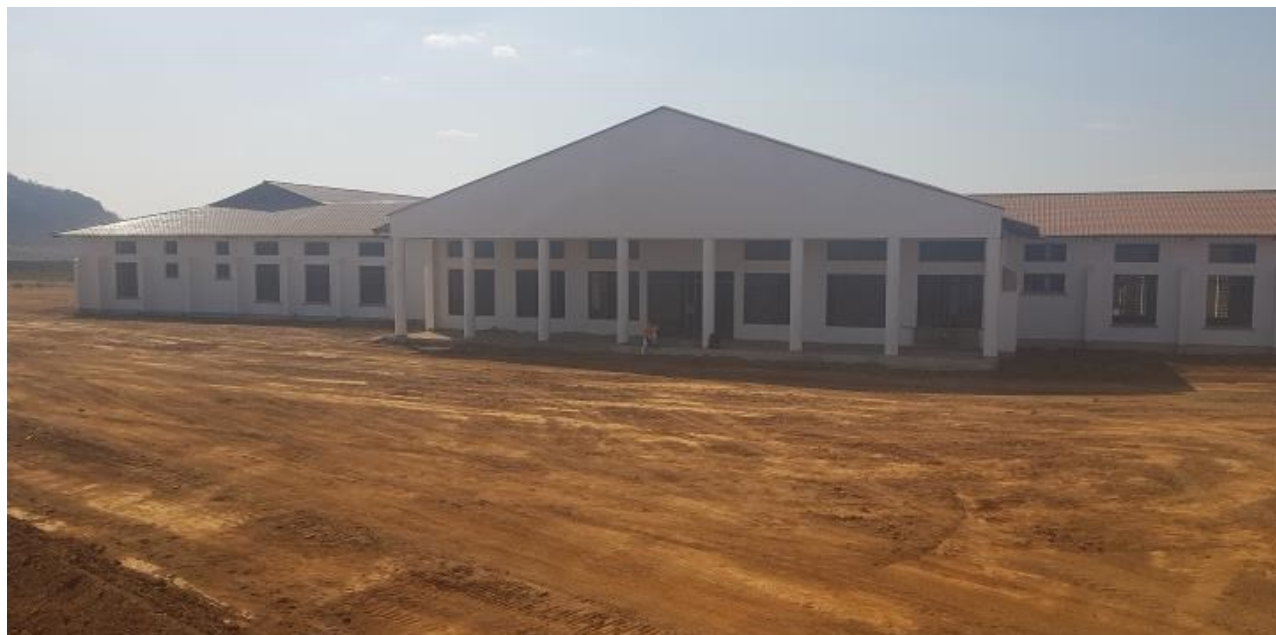
PICTURE 5.1.10—MAIN BUILDINGS AT PHALOMBE HOSPITAL (FINISHING WORKS UNDERWAY)
