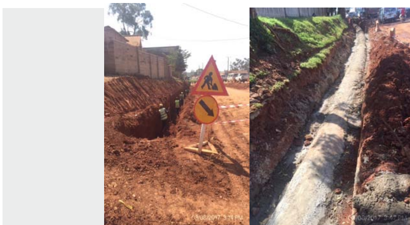
Figure 37: Excavation and Backfilling culvert with mortar
