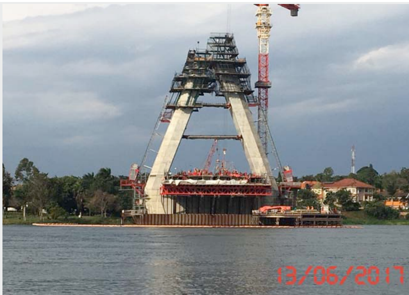
Figure 41: New Nile Bridge under construction
