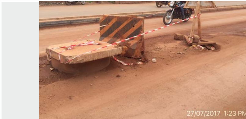
Figure 23: Culvert through the surface
