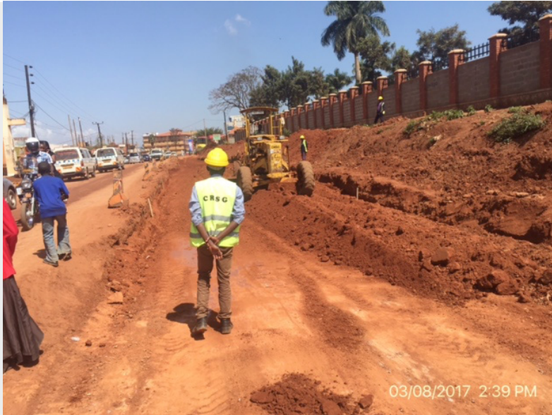
Figure 38: Contractor preparing subbase
