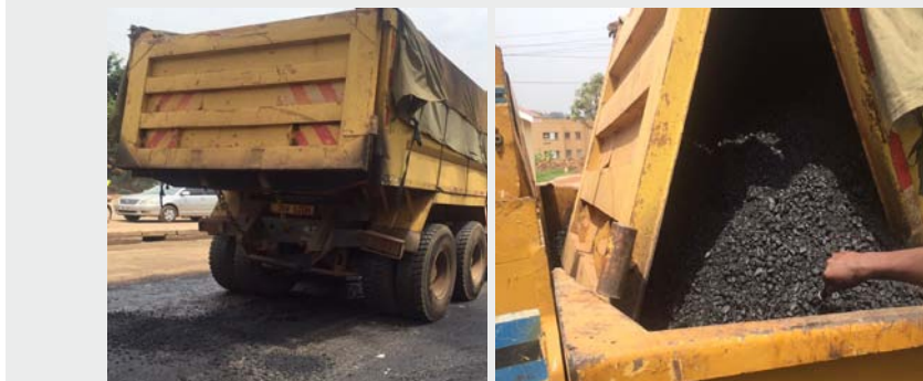
Figure 18: Truck offloading asphalt in the paver
