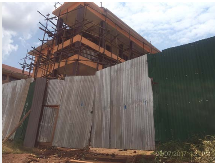
Figure 25: Makerere college block constructed under compensation funds
