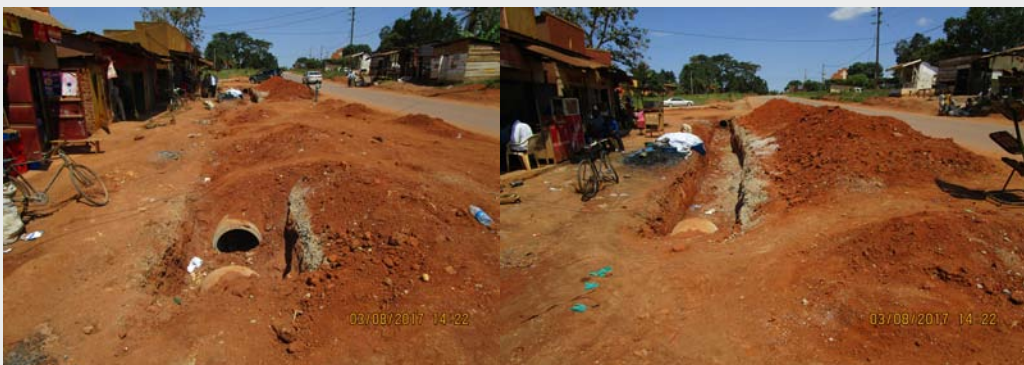
Figure 3: Construction of covered drains in progress along Gayaza road.
