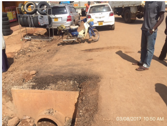
Figure 33: Access road with 2m but with unprotected shoulder
