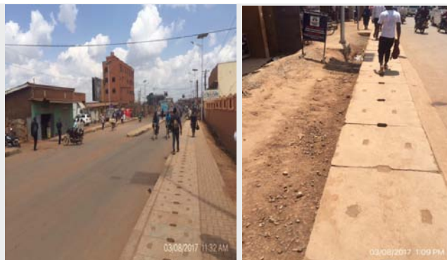
Figure 34: 2m and 1.5m walkway provided
