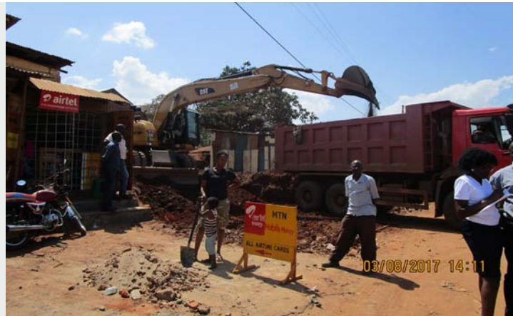
Figure 6: Removal of debris from construction site
