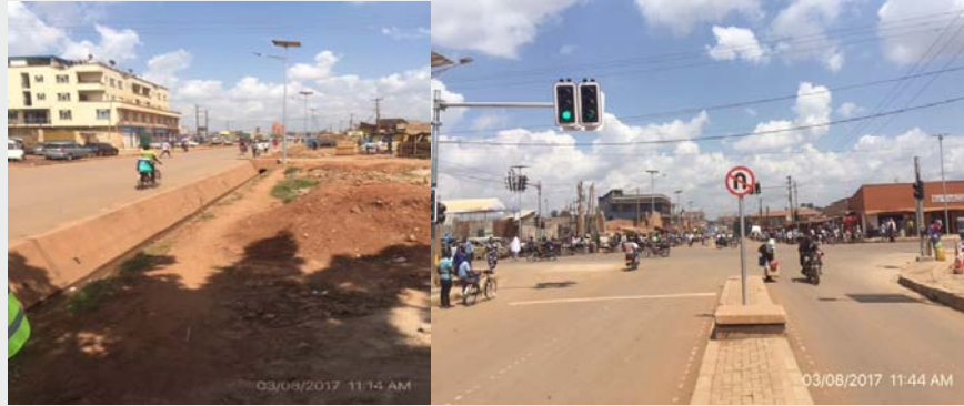
Figure 32: Traffic lights and street lights
