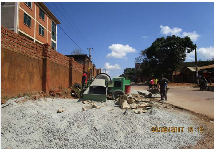
Figure 9: Concrete mixing for concrete works
