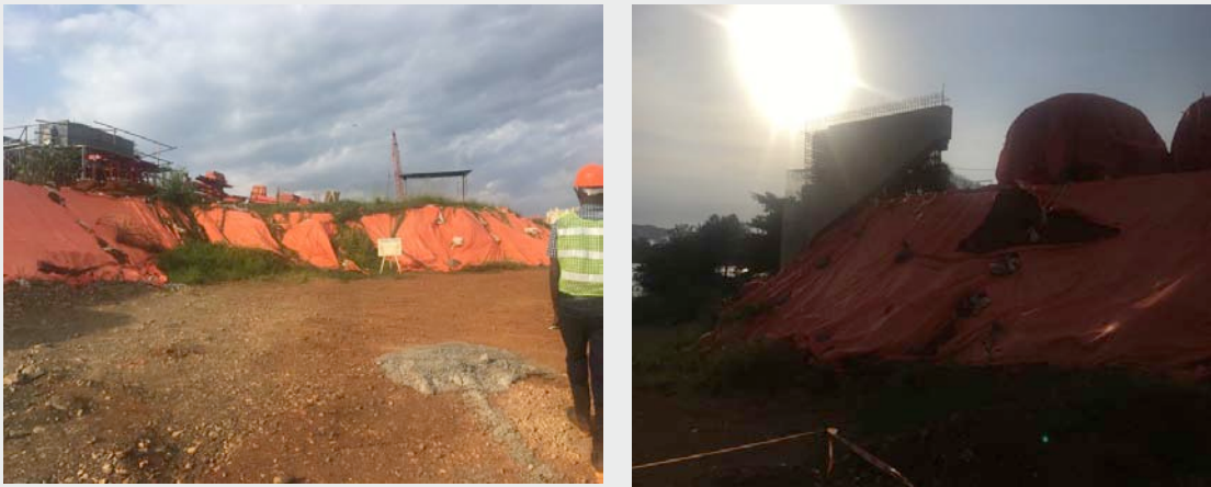
Figure 49: Embankment protection
