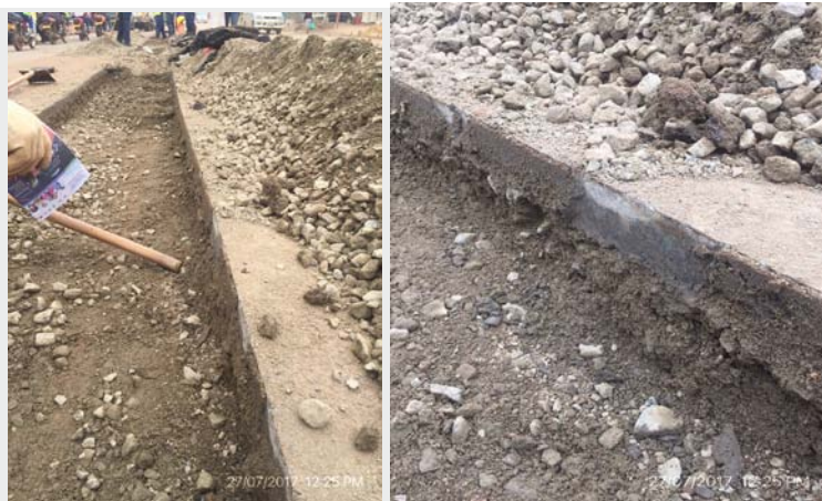
Figure 17: Asphalt Layer thickness (51mm) at km 0+020m
