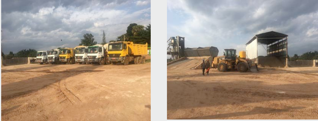
Figure 48: Plant and equipment
