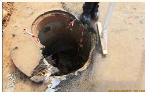
Figure 17: Unsecured service viaduct on St.Noah Nfuufu
