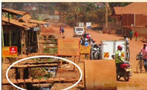
Figure 14: Poorly maintained access at Namasuba road
