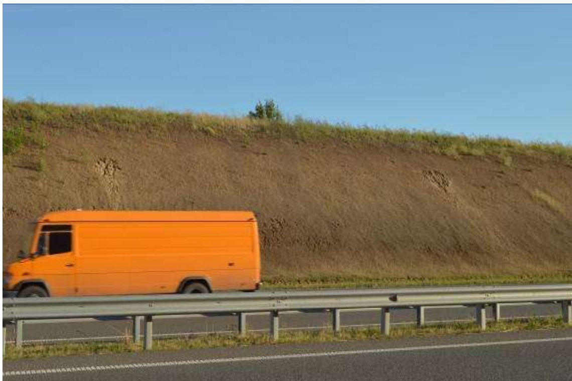
Figure 4 – Erosions, km 311
