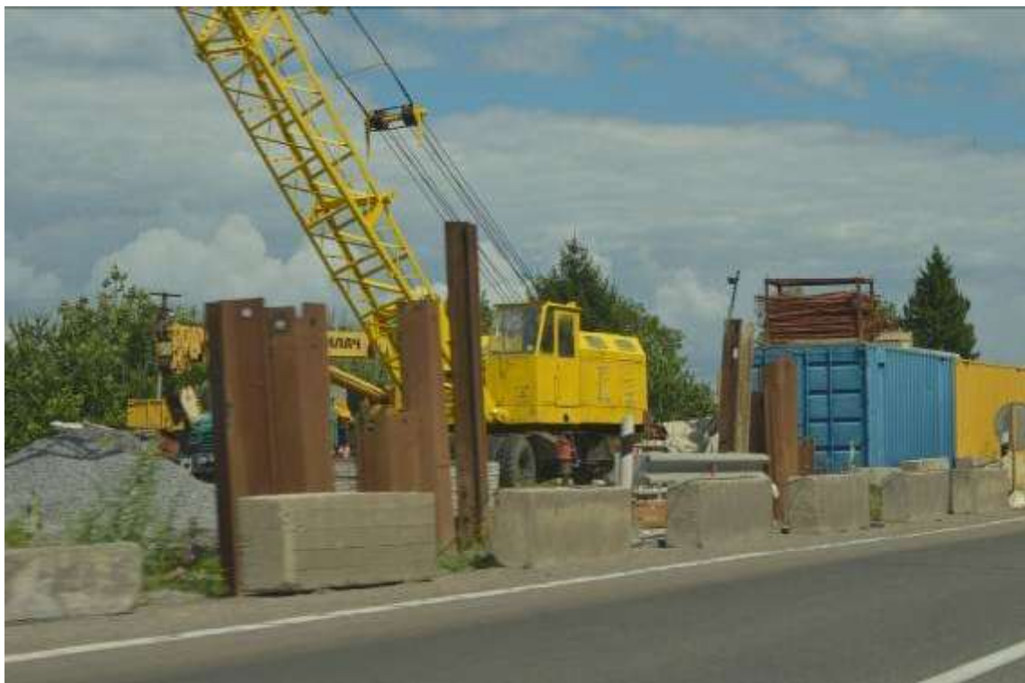
Figure 8 – Construction equipment on construction site
