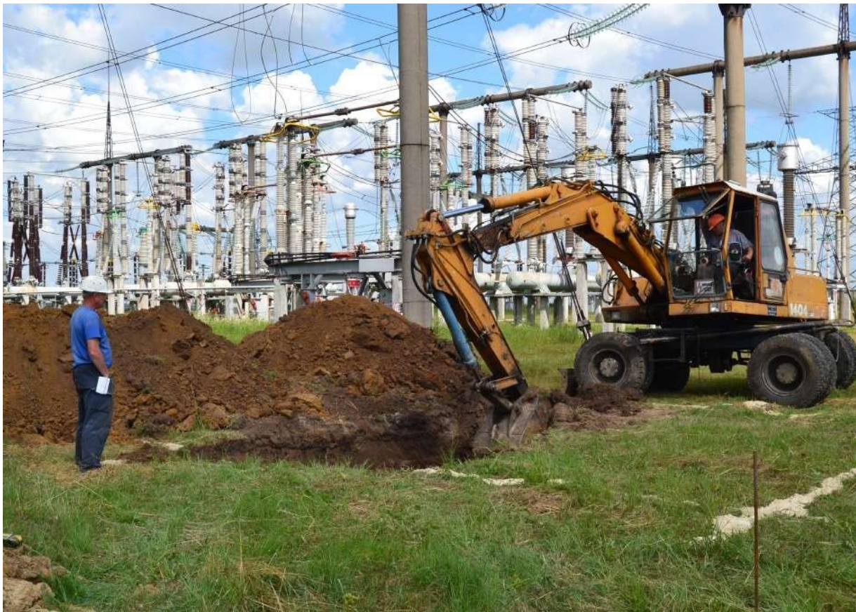
Photo 2: Earthworks for the construction of the foundation for 330 kV portals
