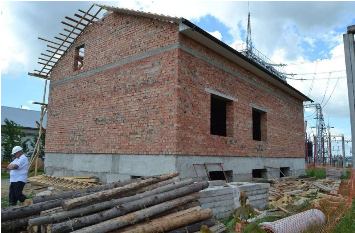
Photo 1: Construction progress of ZPK No. 2, which is behind schedule
