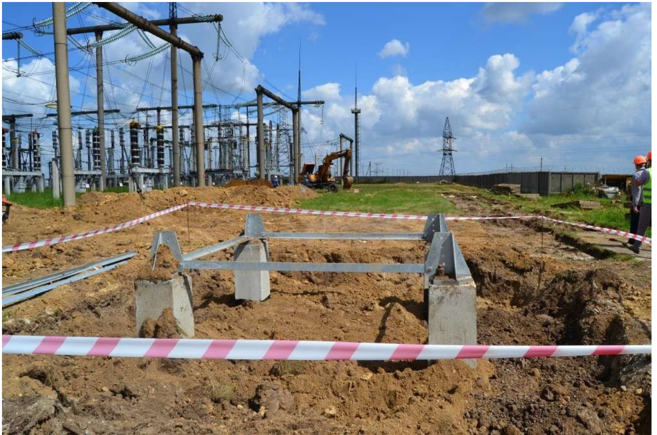
Photo 3: Laying the foundation for the 330 kV transformer portal
