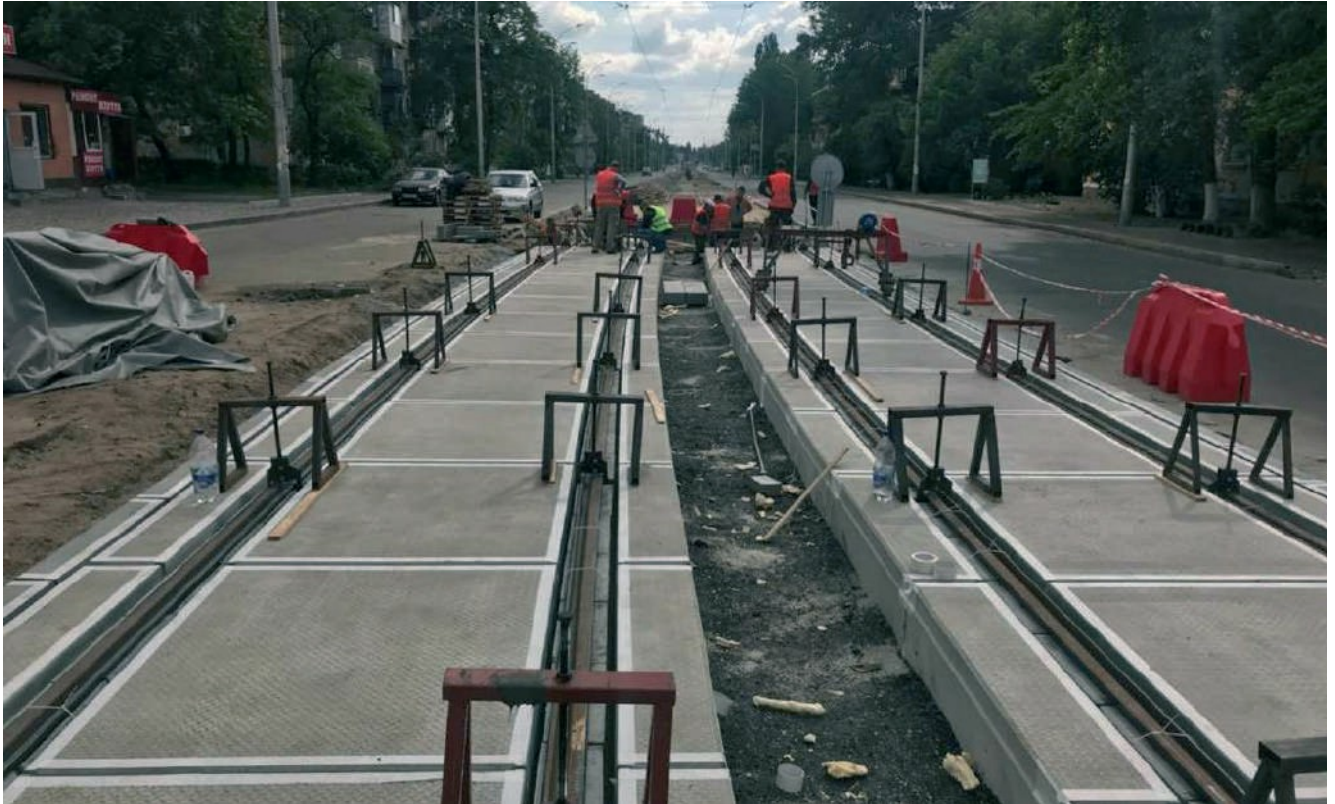
Figure – 60R2 rails are hung and set to the design vertical marks
