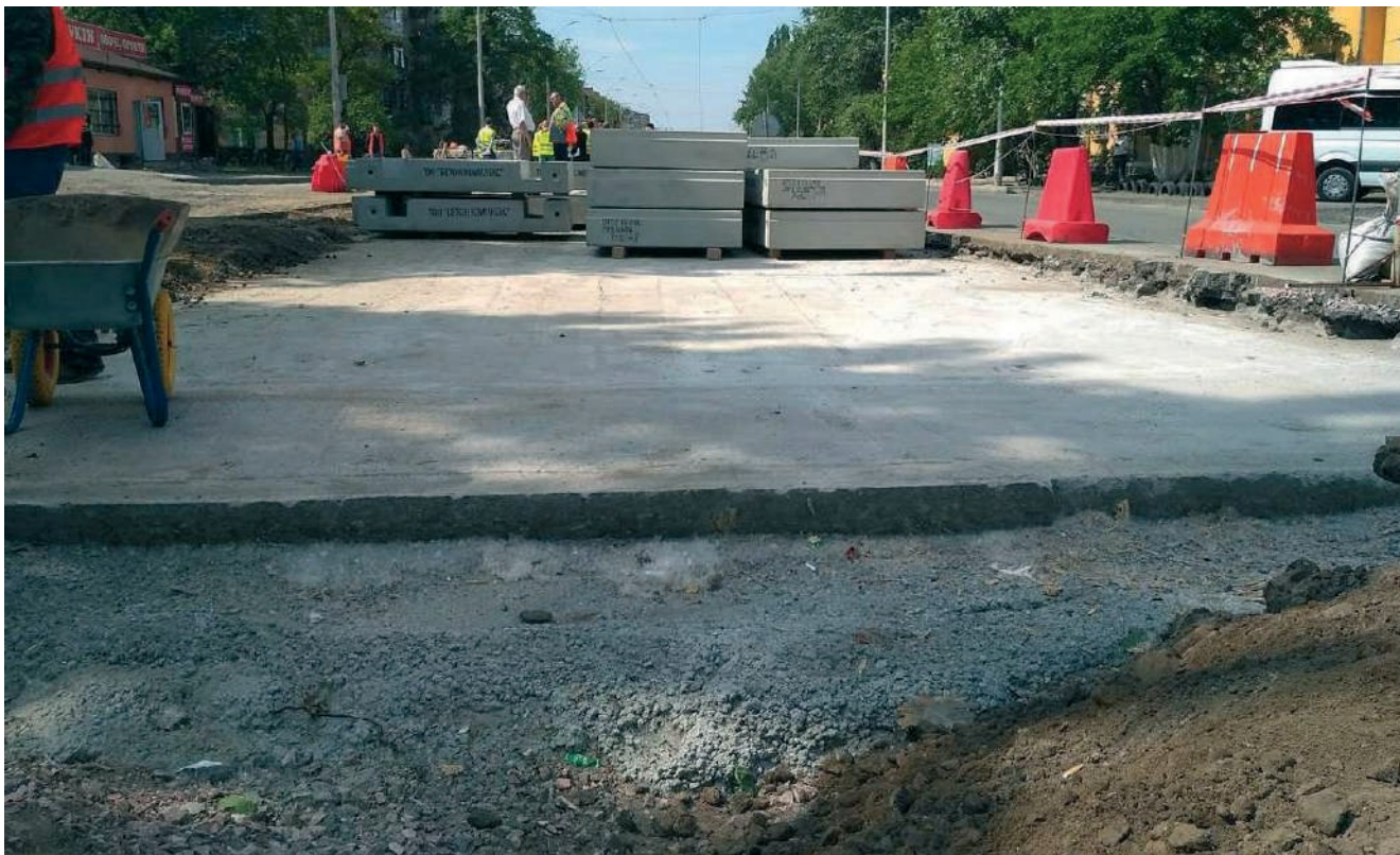
Figure – Installation of a concrete layer in the design of a tram track
