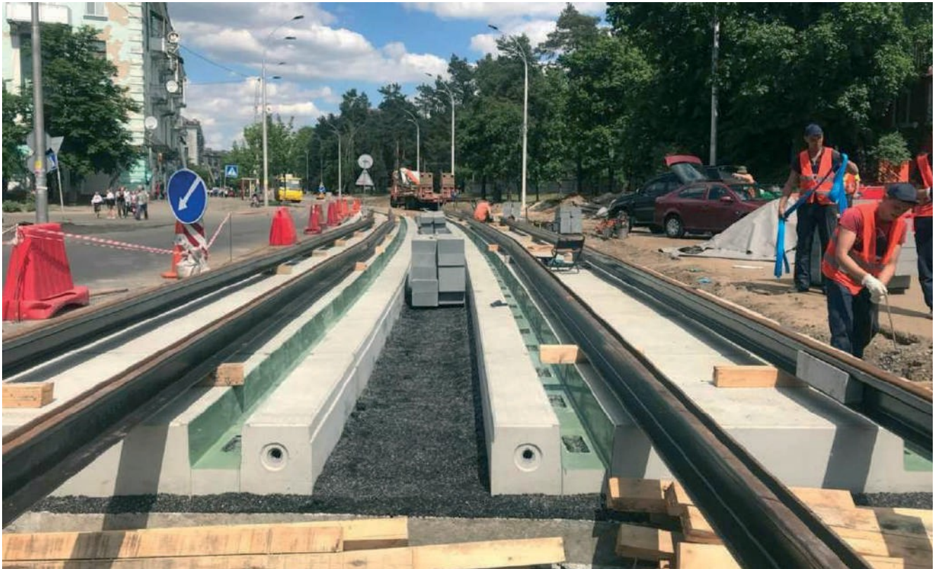
Figure – Repeated cleaning of channel plates and rails, then the rails are cleaned of rust and dirt, degreased, and then primed with a primer
