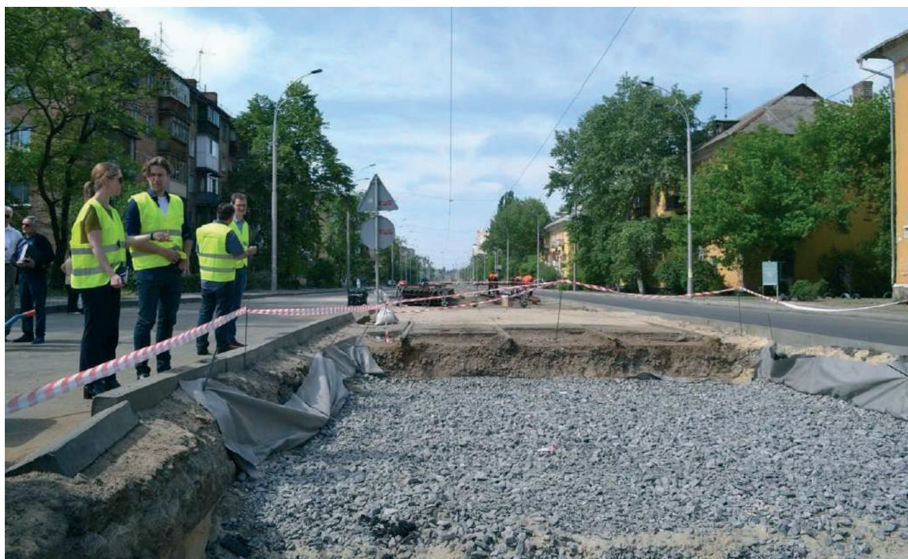
Figure – Installation of Typar SF-49 geotextile and crushed stone layer in the design of the tram track
