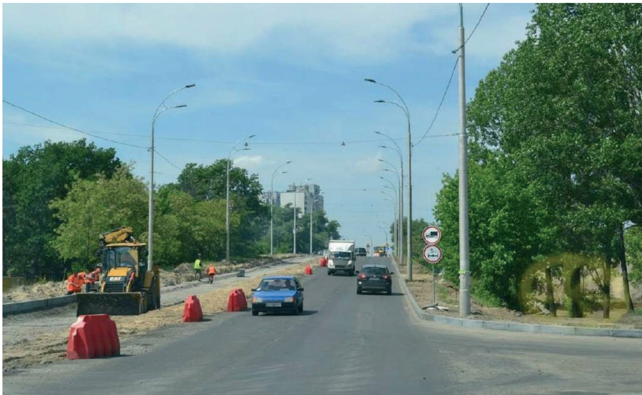
Figure – Section of the motorway after major repairs from PK 6+79.60 (Tractorist Street) to PK 13+58.9 (Manganese Street)
