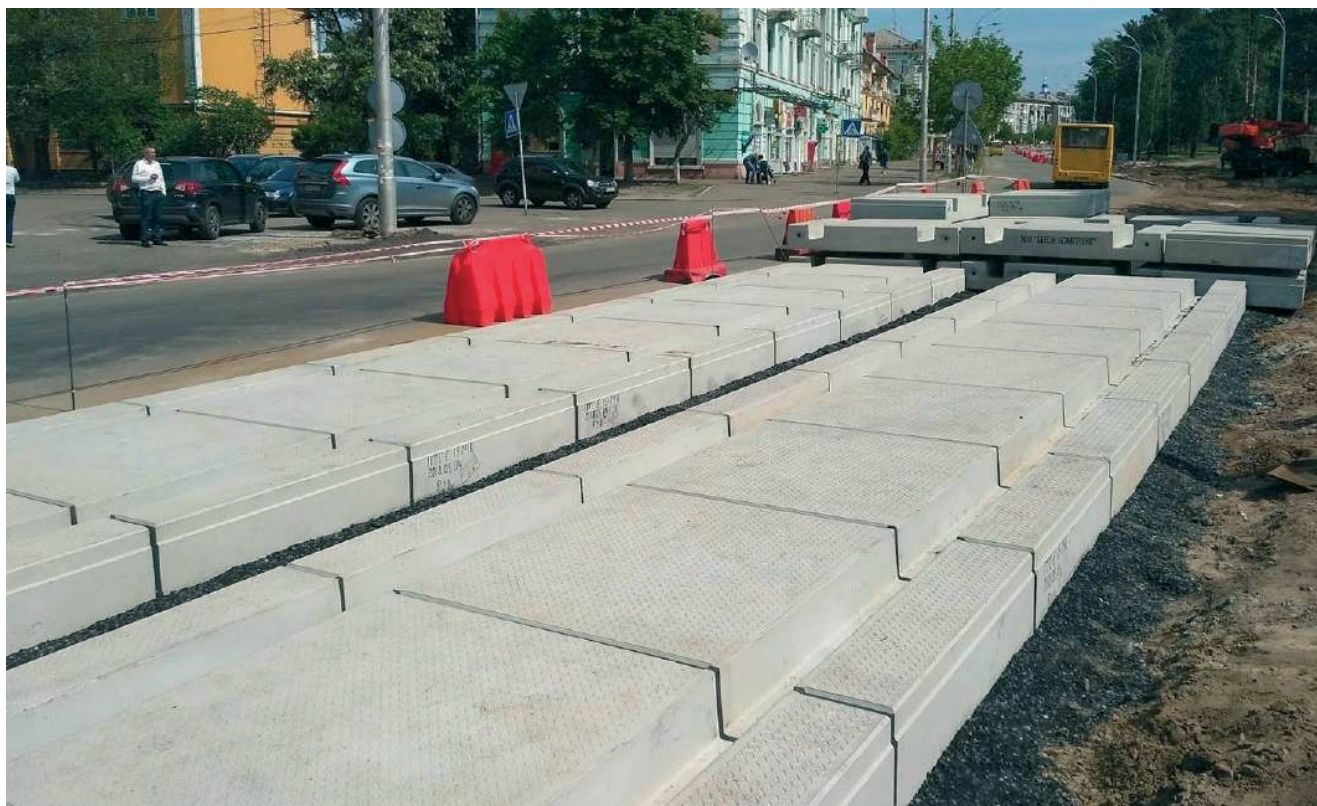
Figure – Installation of block-type tram track with reinforced concrete slabs
