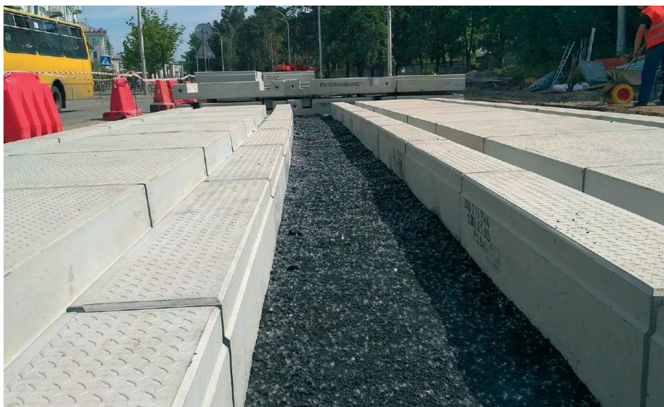
Figure - After laying the geogrid and gradually filling and compacting the crushed stone with a thickness of 120 mm, fraction 40-70 and 80 mm, fraction 20-40 mm, the surface crushed stone cushion is poured with bitumen emulsion (consumption 2.5 l/m 2 ) for better adhesion of fine-grained asphalt concrete with a fraction of 10 mm (layer 3 cm), which acts as a levelling layer and is the base. Installation of a 200 mm thick concrete layer
