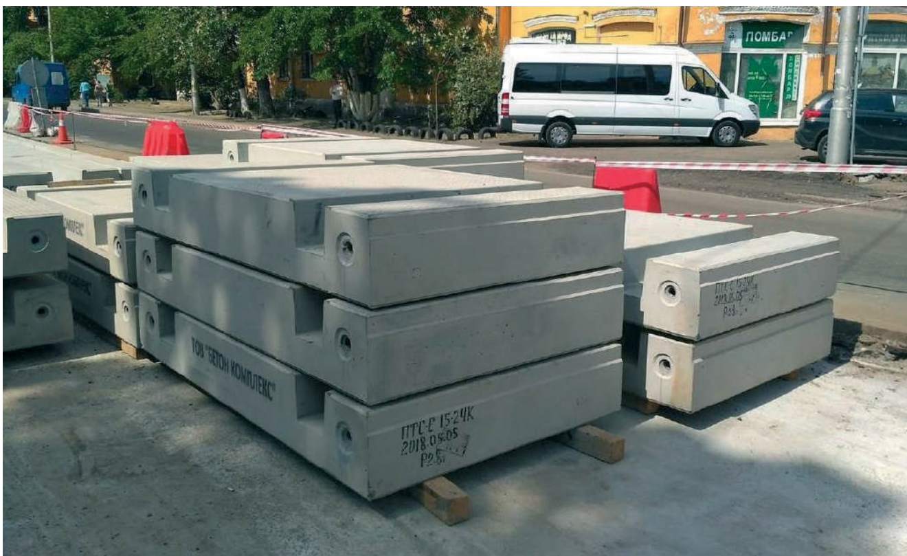
Figure – Reinforced concrete block slabs manufactured by PBK Kovalskaya
