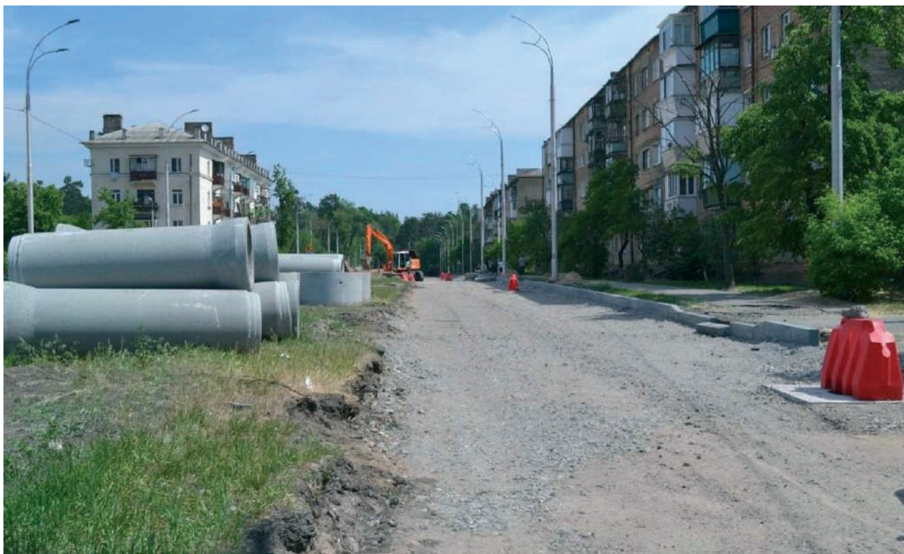
Figure – Preparation before installing KKS-2 type wells
