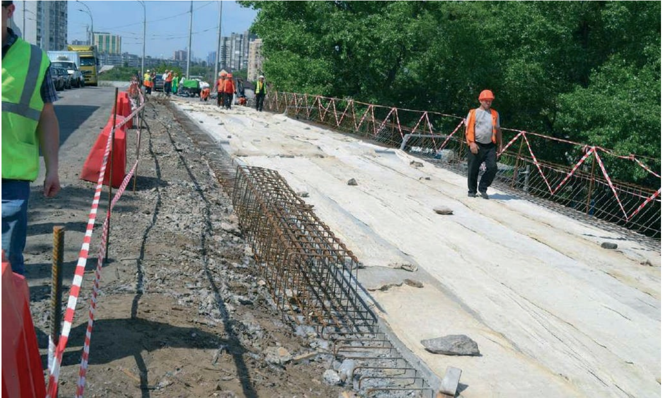
Figure – Strength of concrete in the monolithic reinforced concrete slab of the overpass bridge deck (technological break).
