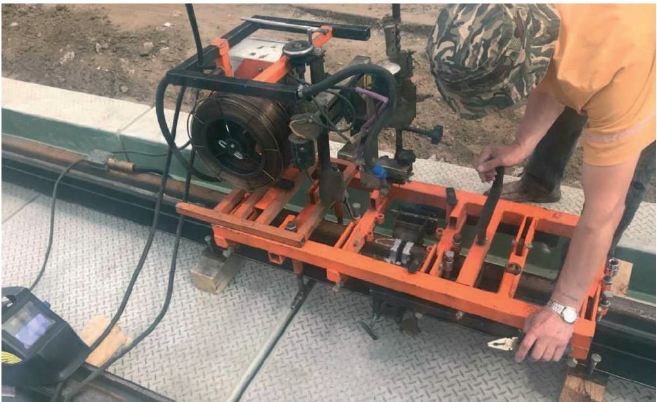
Figure – Welding of 60R2 tram rails together using automated electric arc welding
