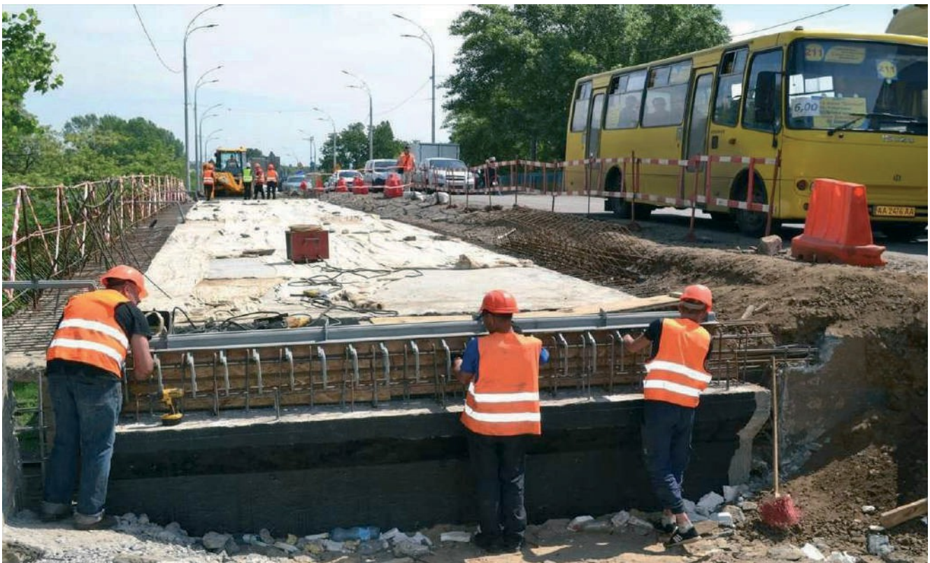
Figure – Installation of a monolithic reinforced concrete slab for the bridge deck of the overpass
