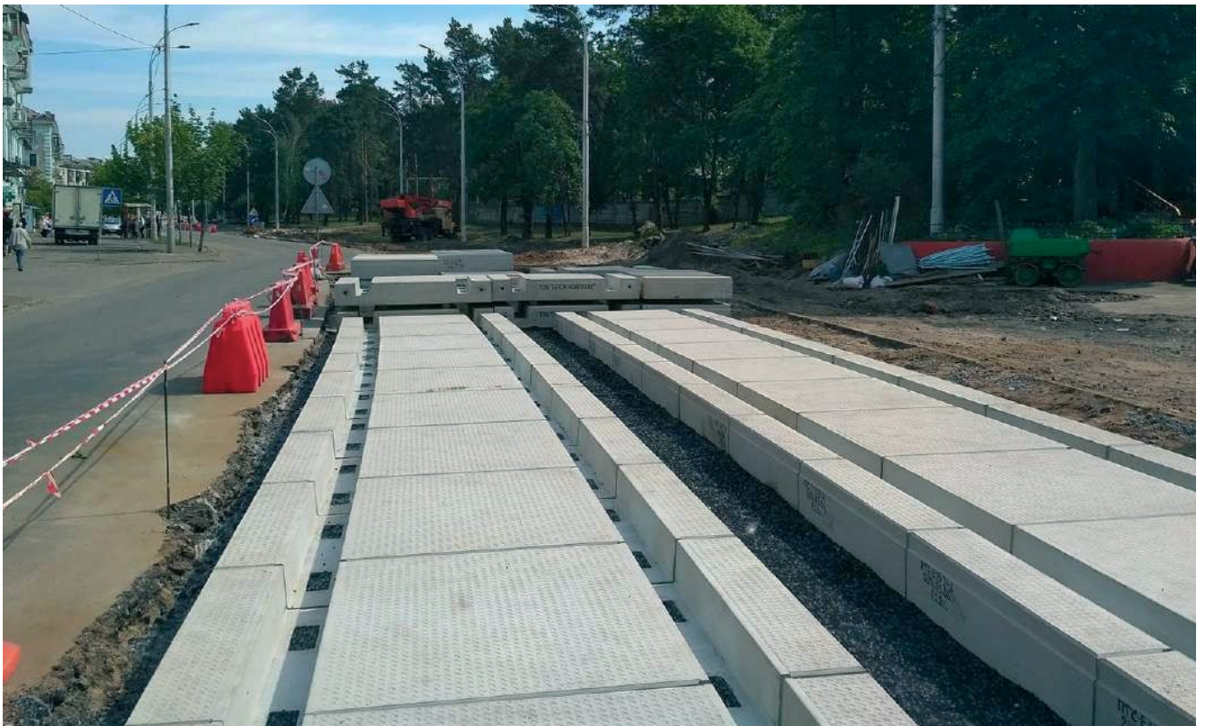
Figure – Installation of block-type tram track with reinforced concrete slabs on Alma-Atynska Street
