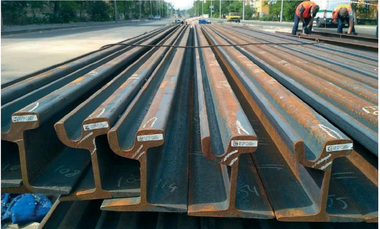
Figure – 60R2 tram rails
