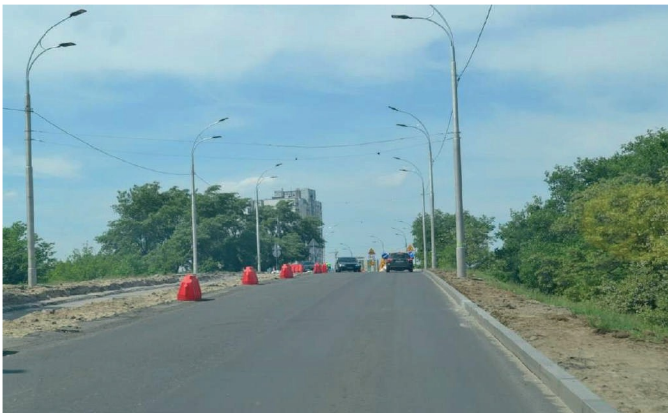
Figure – Section of the motorway at the entrance to the overpass from PK 6+79.60 (Tractoristiv Street) after major repairs
