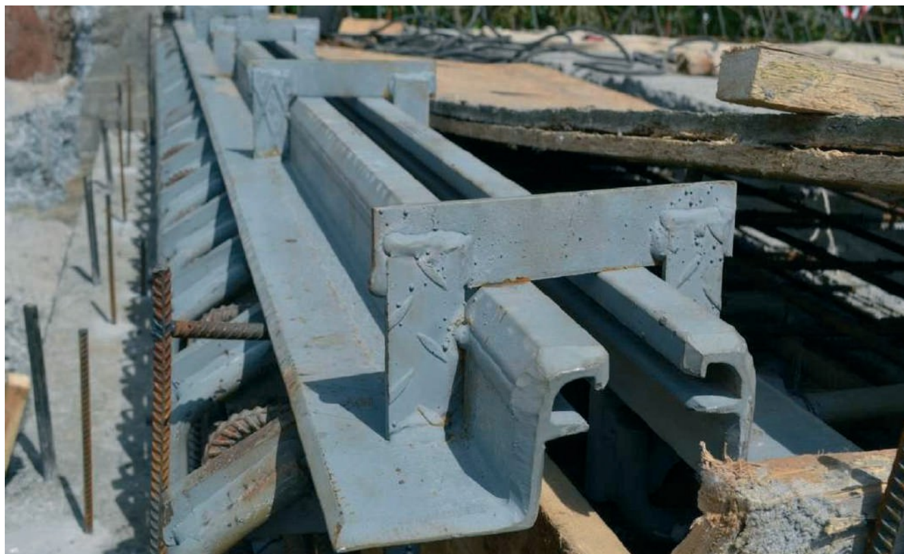
Figure – Completed construction of the expansion joint in the roadway area of the bridge deck (as of 16 May 2018)
